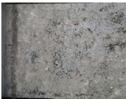
Typical wood-float-finished specimen failure interface profile
