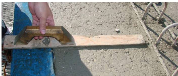
Wood-float finish and the finished surface
