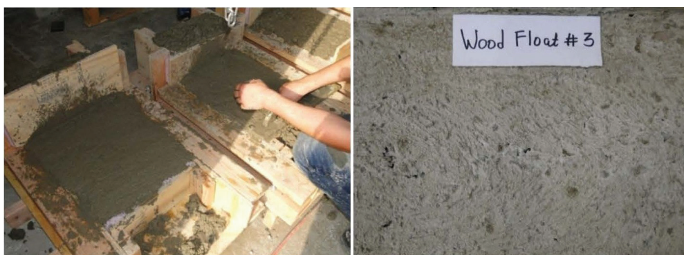
Figure 7. Wood-float finish, showing the preparation process and the resulting surface.
