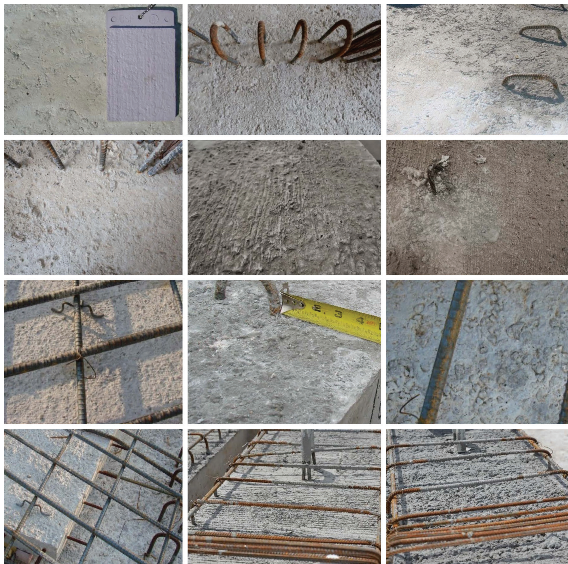
Figure 4. Observed variations in surface roughness produced by Texas precast concrete plants.
