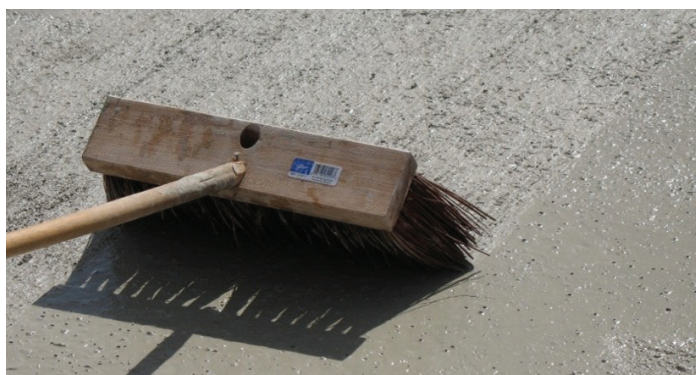
Broom finish and the finished surface
