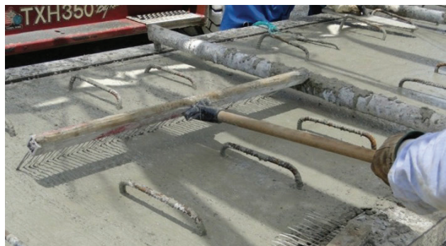
Rake finish and the finished surface
