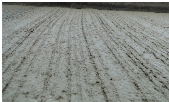
Rake finish and the finished surface
